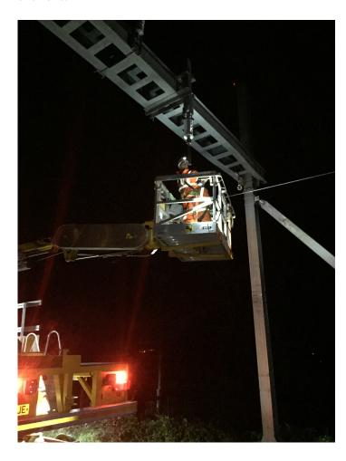
What you're looking at here is the first stretch of new overhead line being installed on the Western Route.
